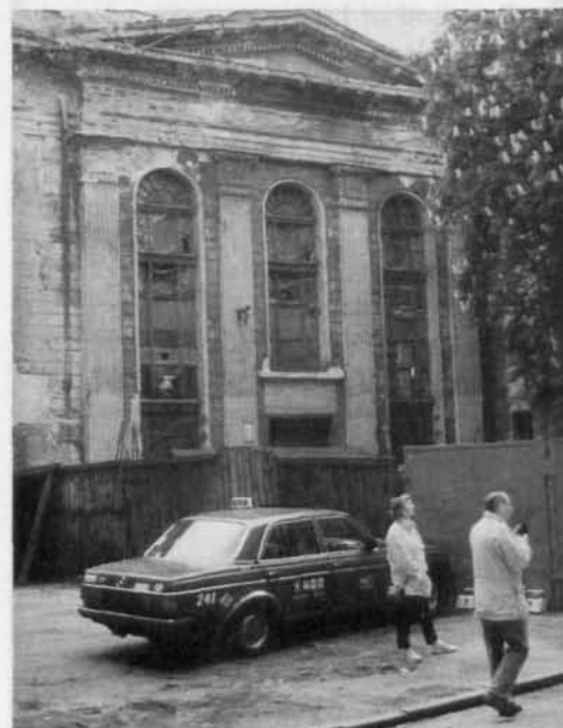
Exterior of the Weisse Storch Synagogue in Breslau, in urgent need of restoration.
