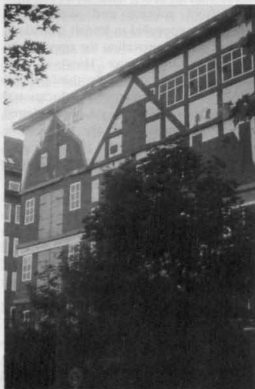
Solid concrete 'Hochbunkers' in Hamburg with houses painted on them to disguise their original function as air-raid shelters.
